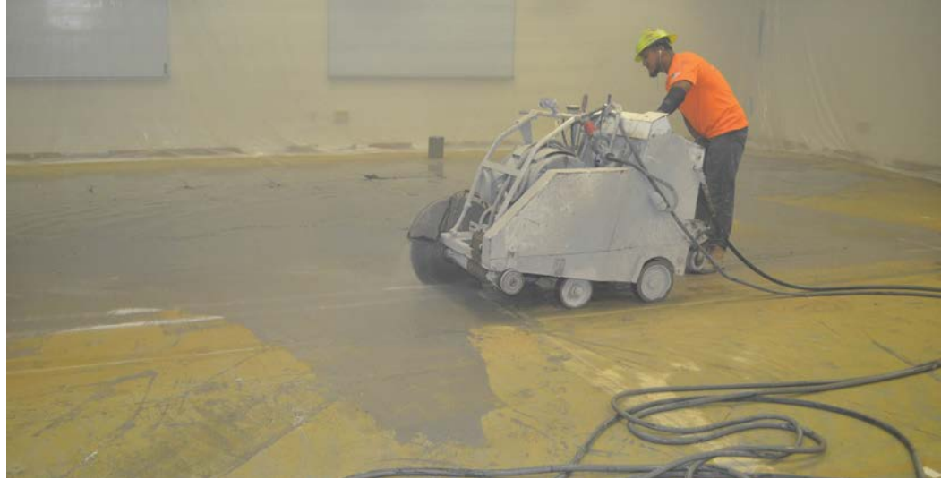
A worker cuts trenches in the CTCPA Education Center's concrete floors to make way for new electrical boxes accessible to all course and meeting attendees.
