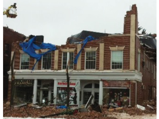
Guilmartin, DiPiro & Sokolowski's Middletown office following its collapse under the weight of ice and snow in 2011, and the rebuilt building as it appears today.
